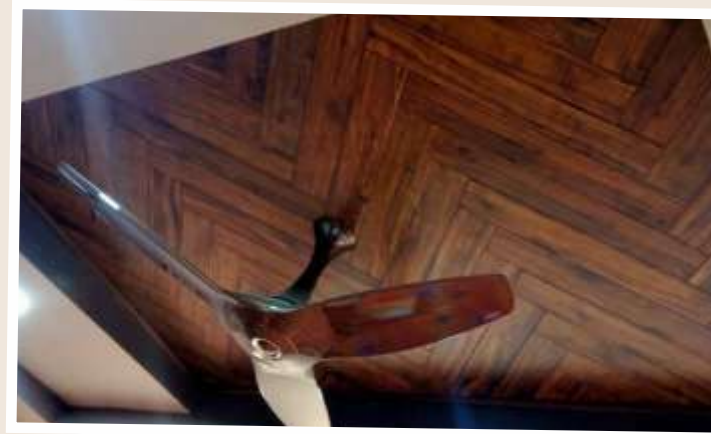
Flooring used in ceiling
